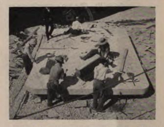
Roof stone 17-1 x 13 1 x 1-6, cut at quarry. Shipped on special car by H, & W. R, R, and built for the purpose.
